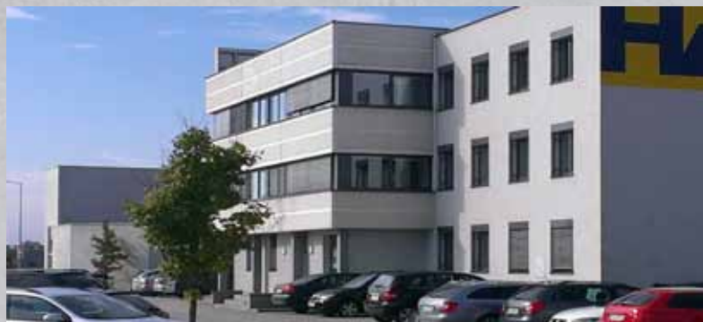
Precast element building facade
